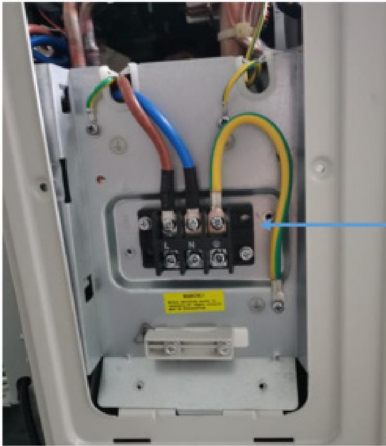
Figure 5-1.4: Power Supply Terminals
